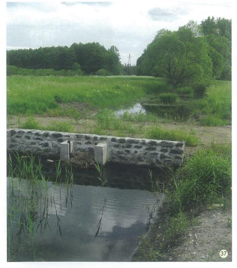
National Park Directorate with the financial support of the EU started nature protection rehabilitation interventions in 2012. The former drainage ditches were dammed by sluices (37) which retained the groundwater flowing into the neighbouring Kígyós Creek. The water driven to the edges of the fen improved the environmental conditions.
