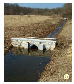
During 2012–13 the Balaton Uplands National Park Directorate with the financial support of the EU carried out rehabilitation interventions. Sluices had been built into the ditches (36) which drove the dammed water into the side ditches and raised the level of groundwater (37). Giant Goldenrod was driven back by mowing.
